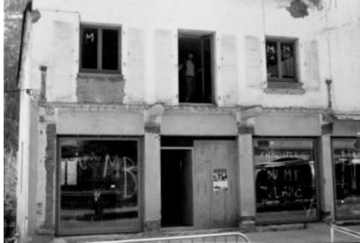
Before renovation of the Chamonix store. Courtesy of Patagonia
